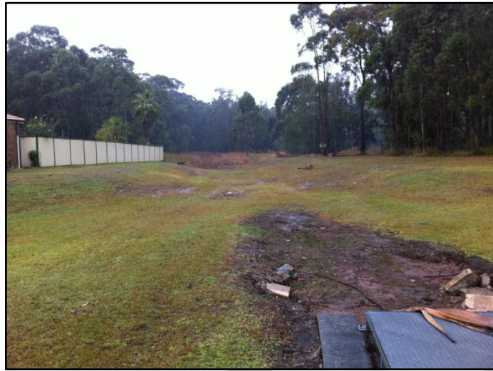
Figure 6-7 Existing Surcharge Structure Downstream of Coachwood Drive
